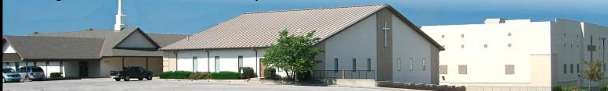
South Haven Baptist Church
